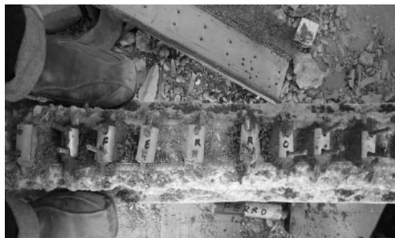
(b) Placement of the connectors in the chiselled beam
