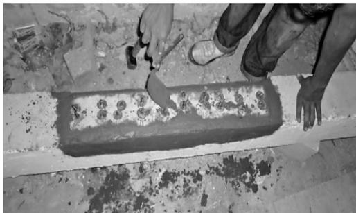
(c) Finishing Surface of beam soffit after fastening Ferrocement Laminates with the connectors
