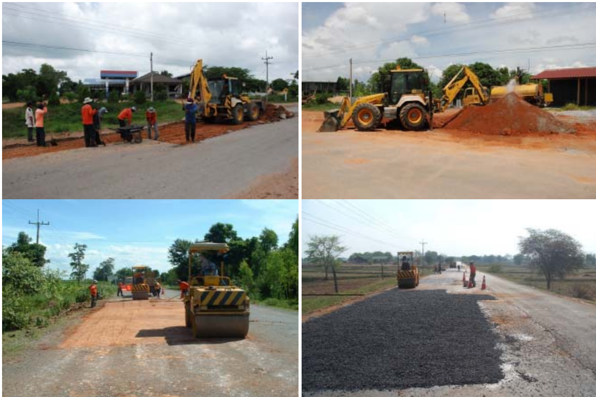
Fig. 11. Pavement maintenance using cement-stabilized lateritic soil
