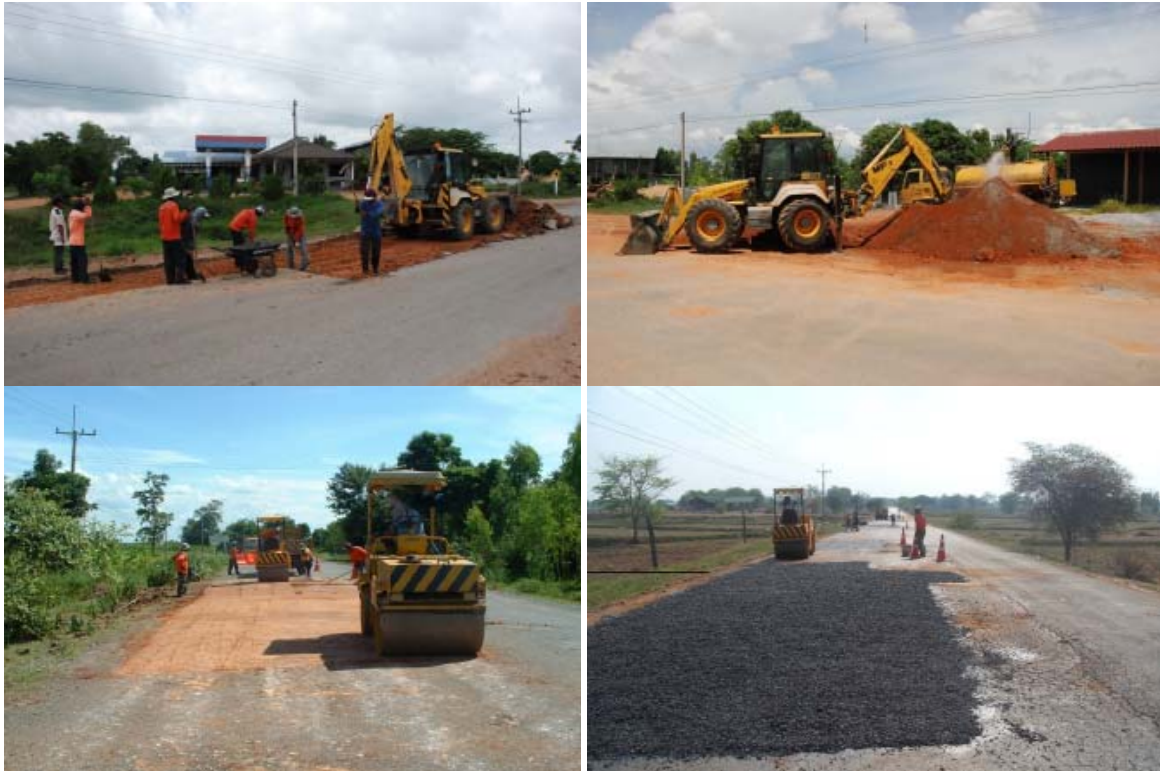
Fig. 11. Pavement maintenance using cement-stabilized lateritic soil
