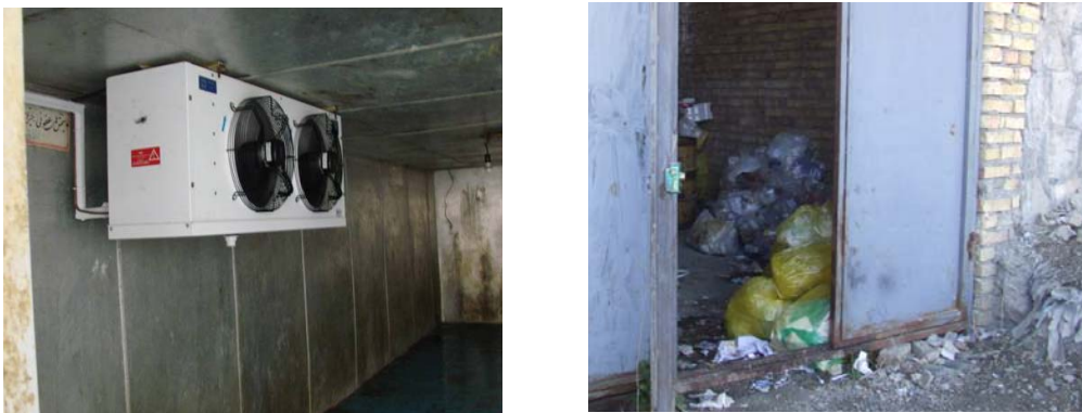
Fig. 1. A storage room with appropriate ventilation and temperature control (left) and a storage room with non-standard conditions (right)
