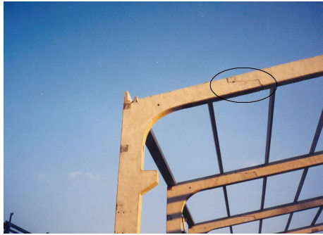
Fig. 1. Scarfed joint of a prefabricated industrial plant
