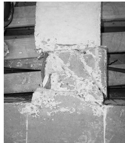
Fig. 11. Observed failure mechanism of specimen RSC1 [12]
