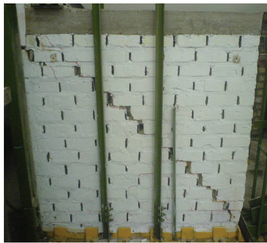
Fig. 7. Mode of failure of the wall NWES
